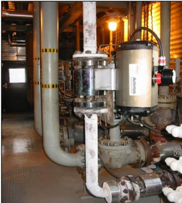
*Figure 2: ValvTechnologies 3" Class 900 V Series valve for molecular sieve regeneration switching installed in July 2003.*
