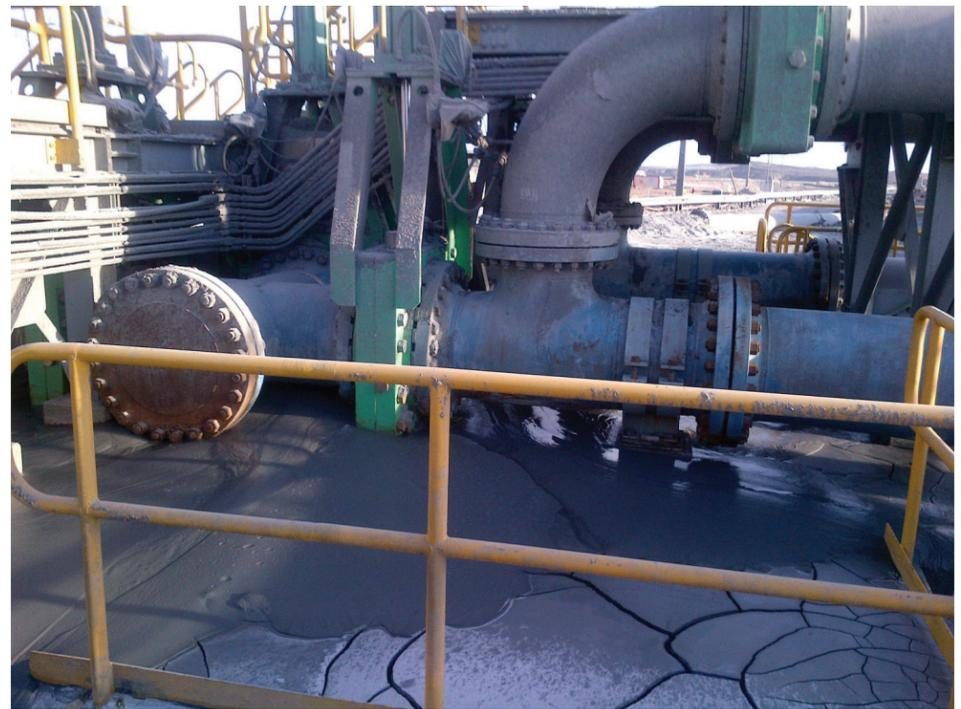
*This discharge from a push-through knife gate is more of an annoyance as it is only seawater and tailings on a tailings disposal pipeline in Chile.*
