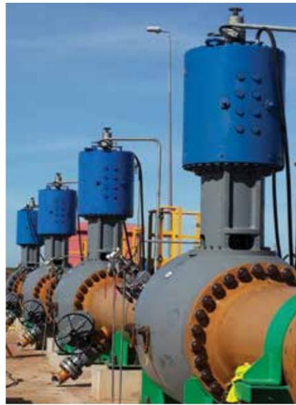
Figure 12: ValvTechnologies Pipeline Isolation Valves for Bidirectional Operation
