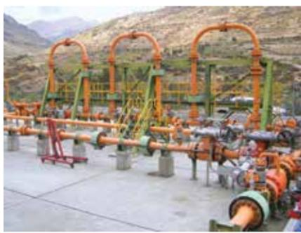
Figure 11: Typical Choke Station with Fixed and Variable Chokes]
