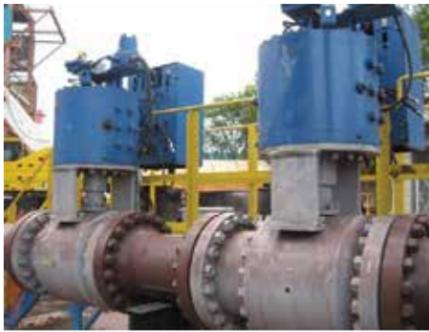
Figure 10: ValvTechnologies Pipeline Station Isolation "Wear and Seal" Arrangement
