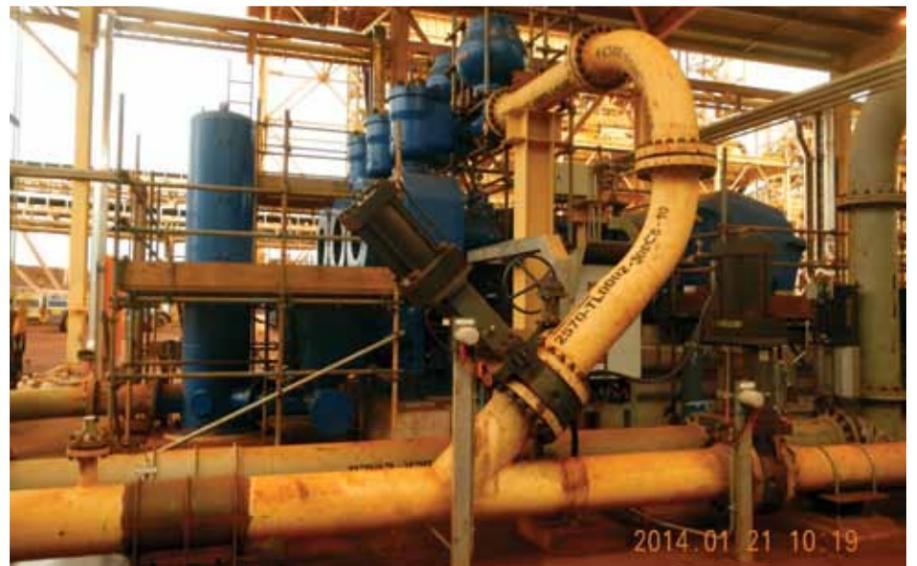
Figure 5: 7 MPa Australian iron tailings system - Class 600 Guided Shear Gates]
