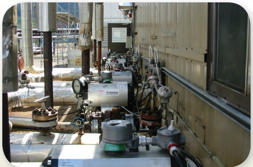
VTI metal seated ball valve in use at gas plant in Northern BC
