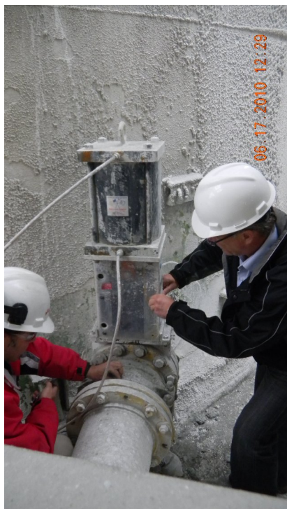
CGIS President Ross Waters shows how to examine the Delta bonnet and adjust the packing.
