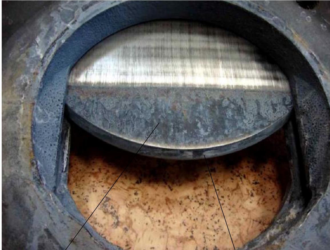
Fig. # 8. Face of the gate at the inlet.
