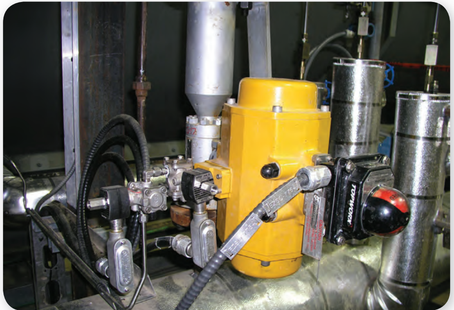
Figure 5: Valvtechnologies V1-1 valve.
